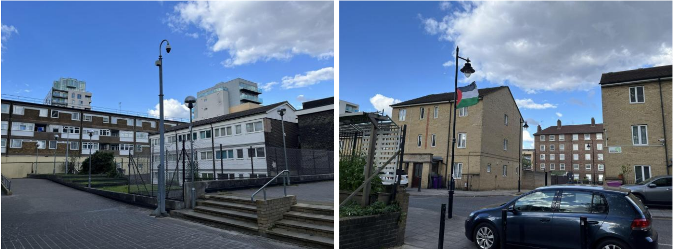
These Tower Hamlets sites are both within easy walking distance of the most economically productive area in the country
